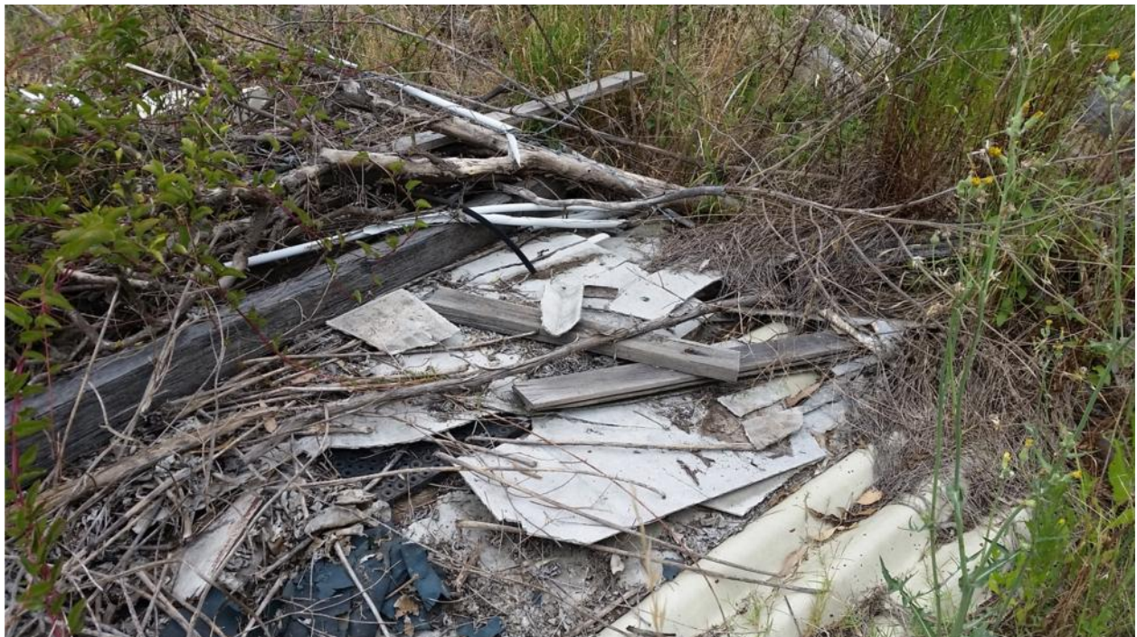
Photo 4: Stockpile of various materials, including possible super-six asbestos sheeting fragments.
