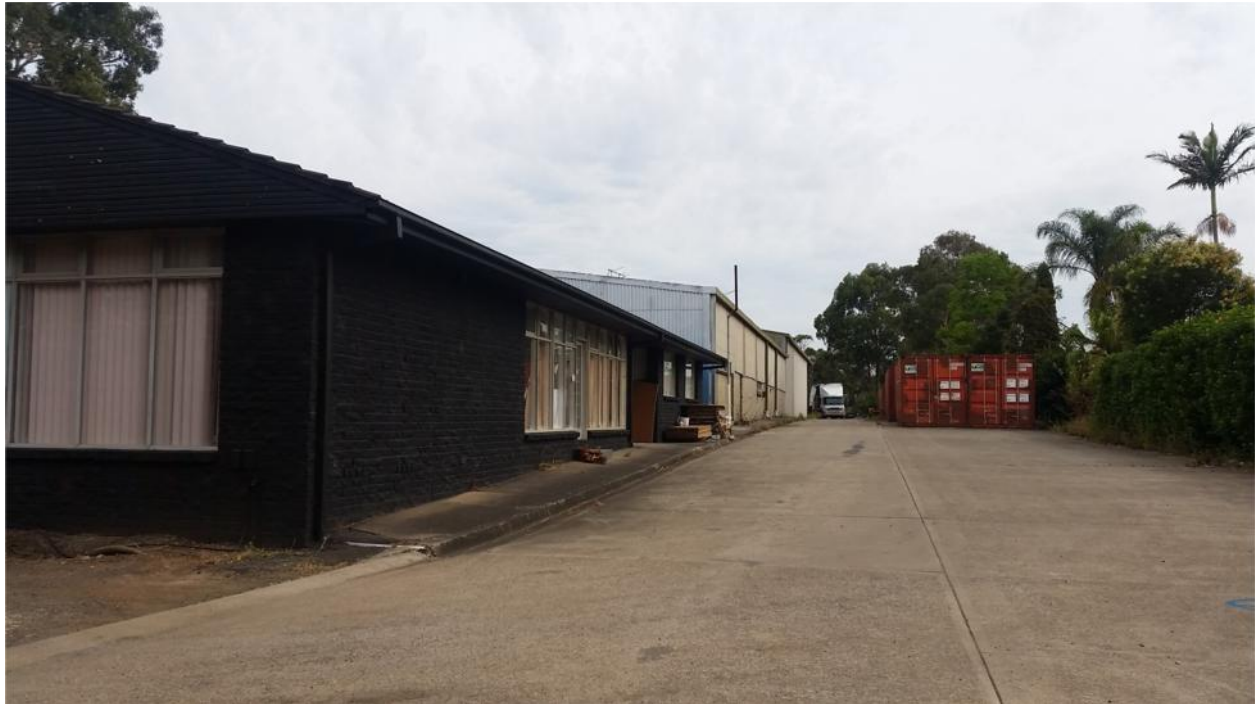
Photo 1: Current site buildings including a former residential dwelling and a large warehouse (photo facing north).
